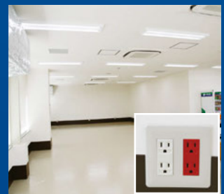
Power outage shelter area (3rd floor) (Red power outlet can be used even during power outage)
