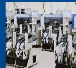
Multiple in-line chip mounters (1st floor)
